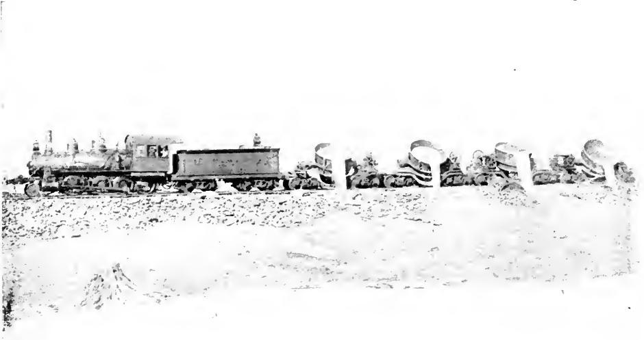
Fig. 76—Pouring Slag on Dump, Canadian Copper Company, Copper Cliff, Ontario.
